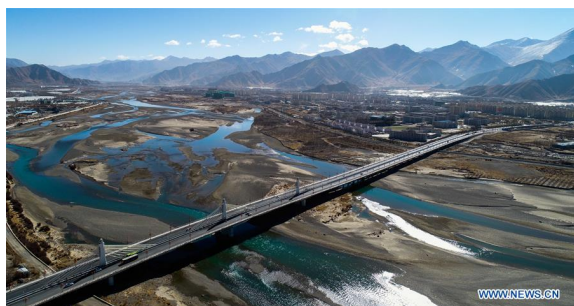
Aerial photo taken on March 4, 2018 shows a newly-built bridge across the Lhasa River, a tributary of the Yarlung Zangbo River, in Southwest China's Tibet autonomous region. [Photo/Xinhua]
