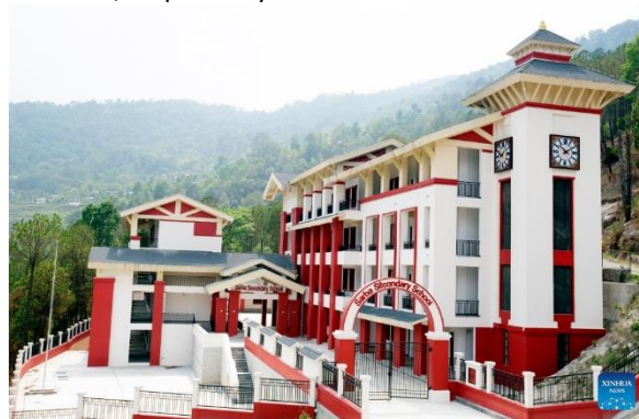
This photo taken on May 15, 2024 shows the newly-rebuilt Sarba Secondary School in Jilu of Dolakha, Nepal.
