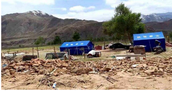
Atsok Monastery's demolition in progress. (Photo: Vera Hue)
