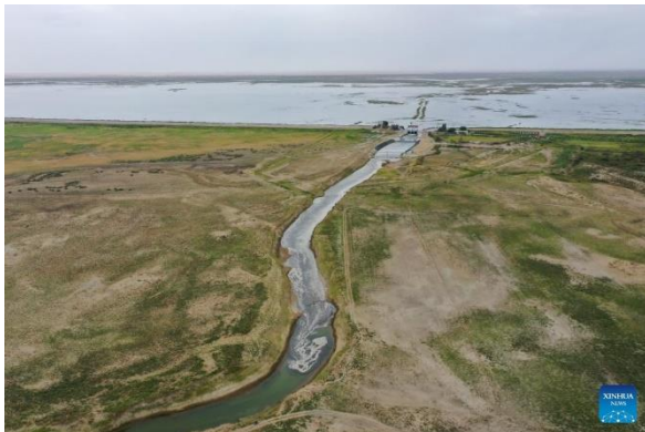
An aerial drone photo taken on Aug. 12, 2024 shows water flowing from the Daxihaizi Reservoir into the river course in Yuli County, northwest China's Xinjiang Uygur Autonomous Region. Northwest China's Xinjiang Uygur Autonomous Region on Monday began discharging water from a reservoir into the Tarim River, China's longest inland river, as part of an ongoing ecological conservation project in the region. (Photo: Xinhua)
