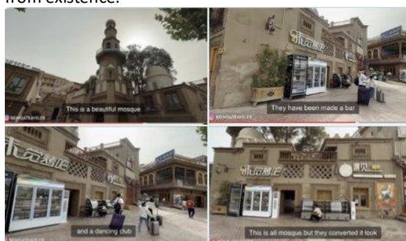
Demolition of 16,000 Mosques in Xinjiang (Photo - X)
