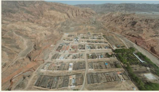
Before demolition began, an aerial view of Atsok Monastery, a 19th century Buddhist monastery located at a bend of Machu river in the Amdo region of the Tibetan plateau. Photo obtained in April 2022, from Tibet Watch
