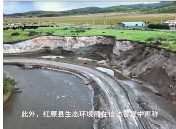
A view of the results of illegal sand and gravel extraction along the Tsaruma River in Kyungchu county, southwestern China's Sichuan province, in an image posted on WeChat by Tibetan resident Tsongon Tsering, Oct. 15, 2024. (Tsongon Tsering/WeChat)
